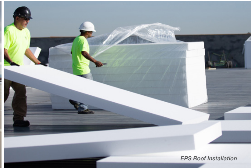
Tapered Insulation Roof Installation
