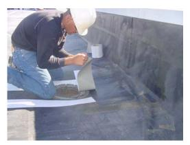
Once all surface areas are completely dry, membrane repairs and seam overlayment can begin with the Coating-Ready Cover Tape.
