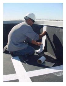
Repeat process for all areas, including vertical surfaces, that are to receive Xtenda Coat coating.
