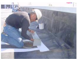
Cut Coating-Ready Cover Tape to the desired length with a utility knife or scissors. Remove release paper backing and press firmly into place, centering tape over cuts or seam overlaps. Remove any bubbles or buckling by firmly pressing with hand or seam-roller.
