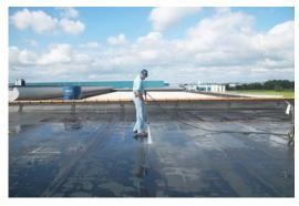
Once at the highest point, work back down to the low point with a final rinse to remove residue from the roof surface.
