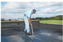
To expedite the drying time and to remove incidental areas of ponded water, squeegee the roof membrane from the high point to the drainage areas.
