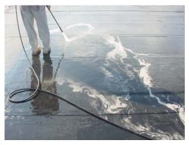
Using a minimum 2000 psi pressure washer, rinse the membrane surface with clean water. Rinsing of the membrane shall begin at the low point of the roof working towards the highest point. The tip of the wand should be held 6-12" above the roof surface when rinsing.
