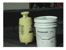
Priming of the roof membrane can take place 24-48 hours in advance of the coating application. Prior to application of the EPDM coating primer, the surface area should be cleaned of heavy deposits of dirt, leaves, branches, and other debris that may have accumulated on the roof surface.
