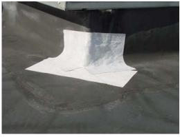
As indicated in the photograph, certain conditions such as curbs, skylights, vent pipes, and other miscellaneous penetrations may require double layers of Coating-Ready Cover Tape to adequately cover repair areas.
