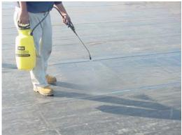
Apply EPDM coating primer with a hand pump type agricultural sprayer. Application is full strength at the rate of 500sq ft per gallon.
