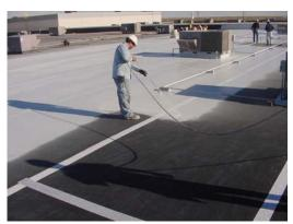
Once the roof area is properly prepared with all repairs completed, application of the Xtenda Coat base coat may begin. Refer to precautions listed in Section 3.04 prior to commencement of coating application. The Xtenda Coat coating must be installed in a minimum of 2 separate applications.
