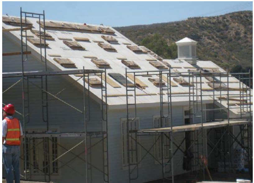
Sure-Board ® Series 200S is the non-combustible alternative for any CFS sheathing application both large and small.
