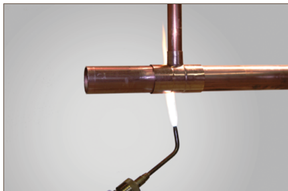
Figure 7.14. Preheating Fitting
