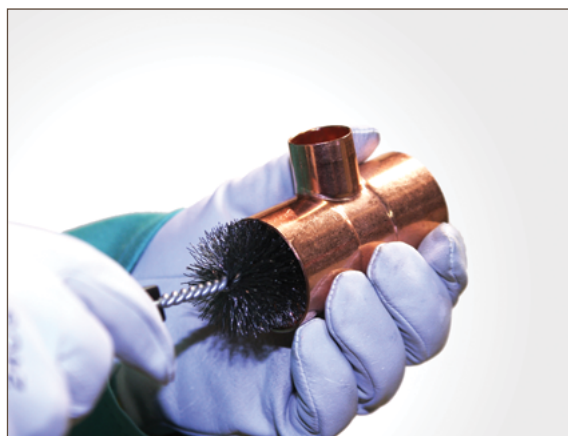
Figure 7.8. Cleaning: Fitting Brush
