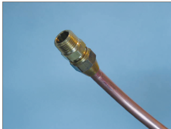
Figure 9.2. Completed Flared Joint
