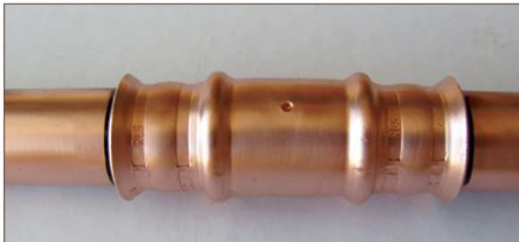
Figure 11.19. Completed joint with insertion marks visible
