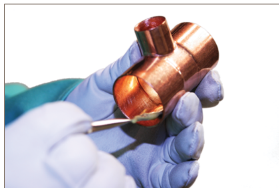
Figure 7.10. Fluxing: Fitting
