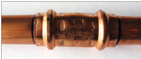
Figure 11.16. Completed installation of a press-connect joint
