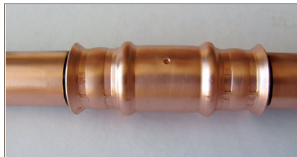
Figure 11.17. Completed joint showing double 360° crimps
