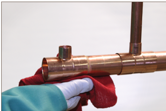
Figure 7.12. Removing Excess Flux
