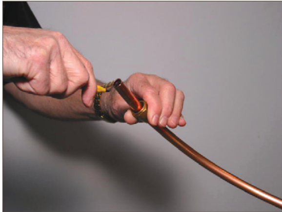
Figure 9.3. Reaming Prior to Flaring the Tube End
