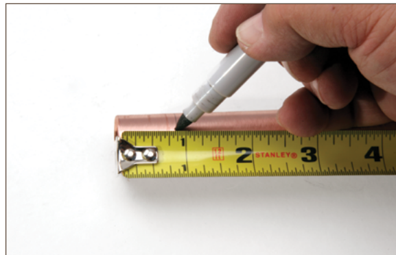
Figure 12.10. Making insertion depth
