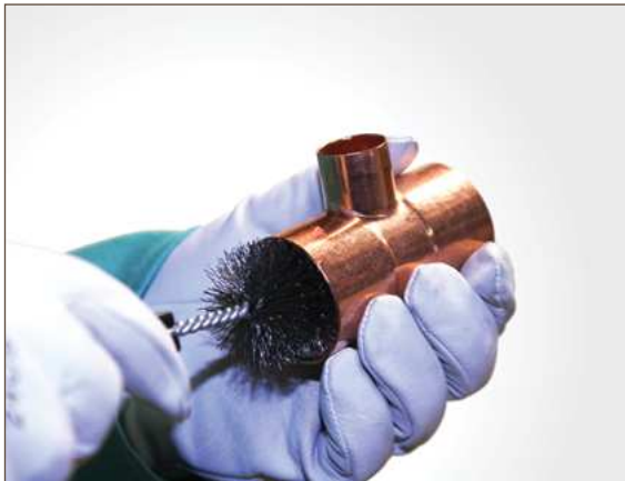
Figure 7.8. Cleaning: Fitting Brush
