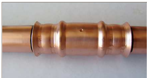
Figure 11.17. Completed joint showing double 360° crimps
