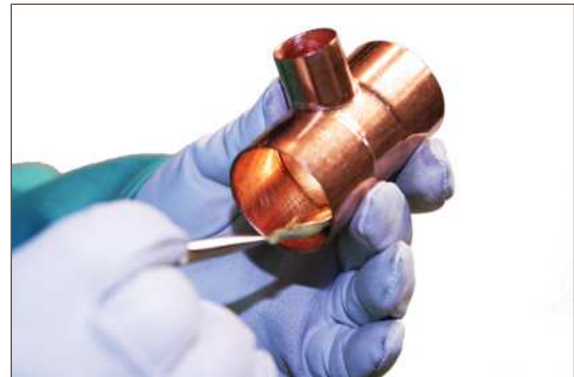
Figure 7.10. Fluxing: Fitting
