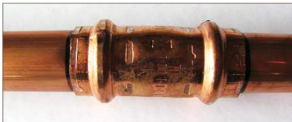
Figure 11.16. Completed installation of a press-connect joint
