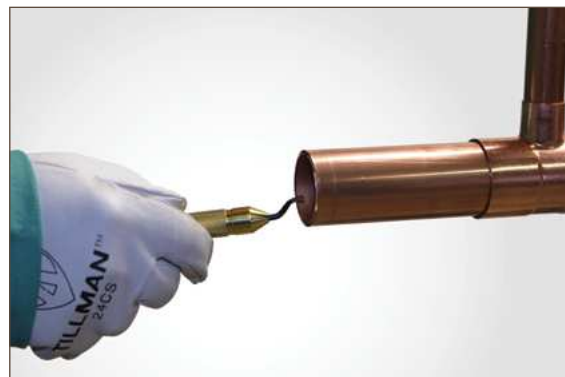
Figure 7.5. Reaming: Deburring Tool
