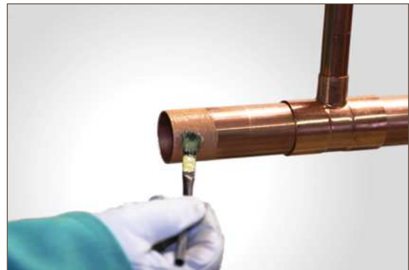
Figure 7.9. Fluxing: Tube
