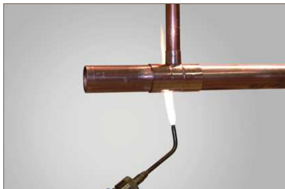
Figure 7.14. Preheating Fitting
