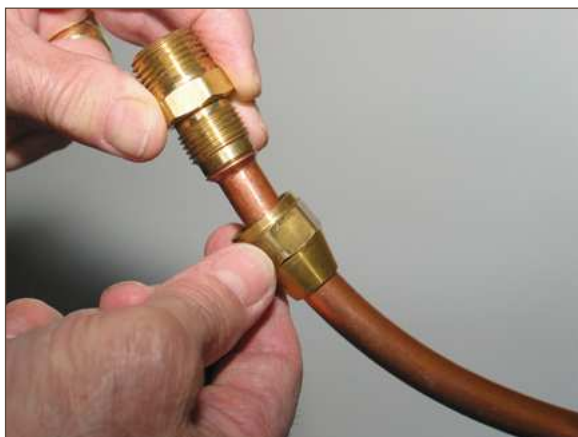
Figure 9.1. Flare Fitting/Flared Joint During Assembly
