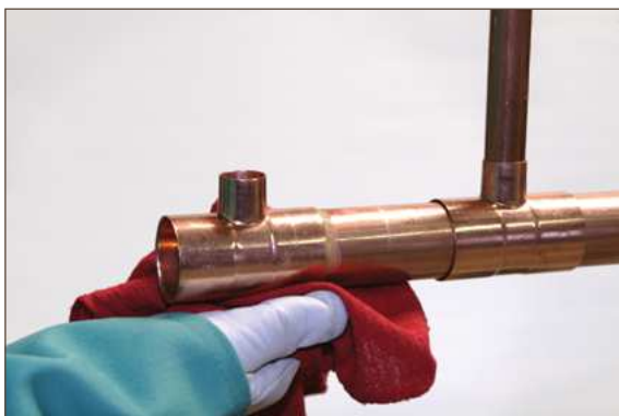
Figure 7.12. Removing Excess Flux
