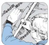
beginning of the cathedral ceiling framing. Work upward until the cavity is filled. Working down the flange, staple about 8" apart until you reach the end of the batt. Do this until the batts reach the exterior walls. Fit batts tightly against each other.
