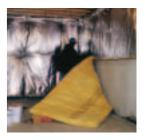
opening dimension between the two rows of furring strips plus 1 1/2." Cut back the insulation 1 1/2" to form a stapling flange at the bottom and fasten.
