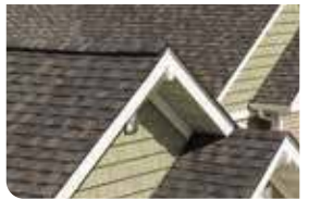
ROOFING AND VENTILATION
