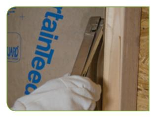
When inset stapling insulation between inclined or vertical framing members, start stapling at the top and work down. Use enough staples to hold the insulation firmly in place (approximately every 8") and avoid gaps and fishmouths between the flanges and framing.
