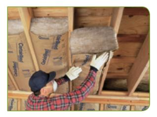
Start installation on one side of the attic, place the insulation between the joists and work toward the center. If necessary, push the insulation under eaves with a broom handle or long stick. If the eave overhangs provide ventilation, be careful not to block the vents and ensure that baffles are in place, as described on page 13.
