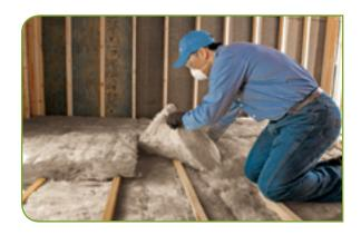
Starting on one side of the attic, place unfaced insulation across the top of joists, perpendicular to the existing insulation, and work toward the center. If necessary, push insulation under the eaves with a broom handle or long stick. If the eave overhangs provide ventilation, be careful not to block the vents and ensure that baffles are in place, as described on page 13.
