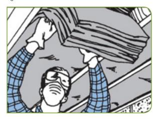
If the insulation completely fills the joist space, one of two methods can be used to hold it permanently in place:
