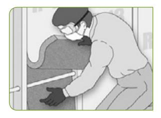
Split insulation to fit around electrical wires and pipes.
