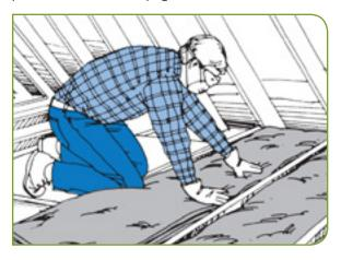
When using insulation batts, place them one after the other until you reach the center. Simply cut the insulation to fit. Install insulation the same way on the opposite side of the attic, working from eaves toward center.
