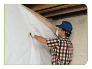
Basement Wall Blanket Insulation is used in semi-finished or unfinished residential and commercial basement areas. It is installed horizontally either in half-wall or full-wall applications (requirements depend on local building code — check with your local building official). For full installation details, please refer to the Basement Wall Blanket Insulation Product Spec Sheet (30-45-052).
