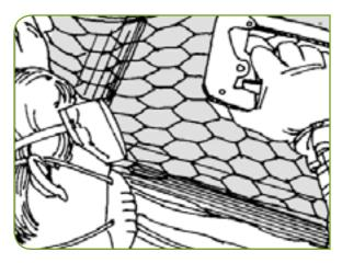
Wire lacing. Galvanized, malleable wire may be laced around nails protruding from the faces of the joists or the wire may be stapled to the joists. Space the wire and nails as needed to prevent the insulation from sagging.
