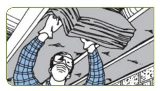
When installing insulation in floors that are not as thick as the joist depth, the insulation must be pushed up firmly against the subfloor so there is no air space between the top of the insulation and the subfloor that will allow heat to be lost at outside walls. In this case, the insulation should be secured in place with:
