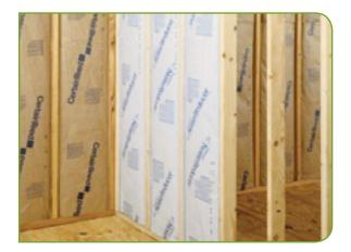
The key areas to insulate are exterior and interior sidewalls, ceiling/floor assemblies and the perimeter of any room addition. Interior walls are especially important to insulate in order to keep noise from traveling between rooms.
