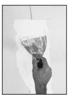
Torn face paper. Peel away any loose paper. Apply a very thin layer of joint compound, using a finishing knife large enough to cover the damaged area. Feather it to get a smooth finish. Let it dry for 24 hours and apply a second coat, if needed.
