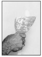
Popped nails. Press the board firmly against the framing member. Drive and dimple a new nail about 1- 1/2" from the popped nail. Then drive the first nail below the surface of the board. Cover the dimples with joint compound.
