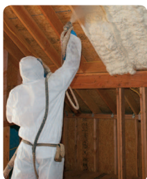
Spray Foam Insulation
