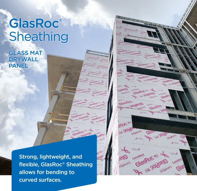
GlasRoc Sheathing and GlasRoc Sheathing Type X are weather resistant drywall sheathing panels consisting of a non-combustible gypsum core and fiber glass face and back mats, designed to provide exceptional mold and moisture resistance for exterior sheathing and soffit applications.
