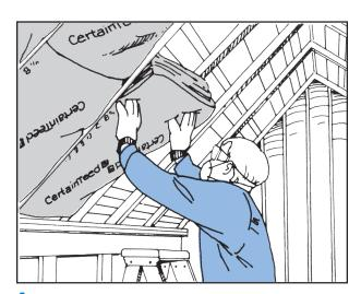
Fit the end of the batt snugly against the top plate of framing at the beginning of the cathedral ceiling framing.
