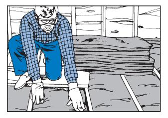
Start installation on one side of attic and work toward center. Push insulation under eave with long stick. If the eave overhang provides ventilation, be careful not to block the vents.
