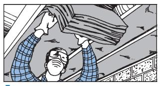
Place insulation between the floor joists. Start at one end and work out. Insulation will stay temporarily. If faced insulation is used, the vapor retarder should face toward the heated area of the home and be in contact with the floor above.
