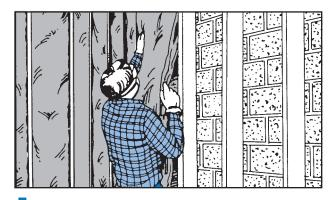
No stapling is necessary. Once the framing strips have been applied, just fit batts between strips.
