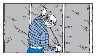
**2** If required, cover with a vapor retarder for installation over framing strips. Do not leave exposed. Cover with an approved material such as gypsum board.
