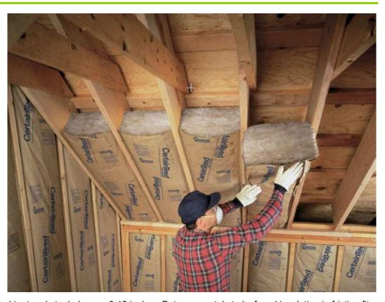
and is then meant to be pulled taut and stapled every 8-12 inches. Between metal studs, faced insulation in friction fit, and stapling flanges should be folded in, or SpeedyR™ tabless batts should be used.
