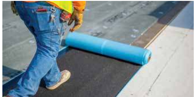
Vapor Retarder Installation
