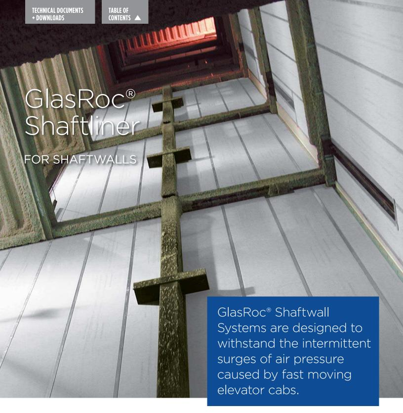
Gypsum shaftwall systems have replaced traditional masonry for interior vertical enclosures like mechanical and elevator enclosures, stairwells, and other mechanical chases. GlasRoc Shaftliner is ideal for use in commercial shaftwall systems, delivering lightweight construction, thinner walls, easy installation and clean up, and cost-effective construction.
