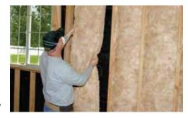
energy in the residential and commercial new construction, remodeling and reinsulation markets. In addition to its thermal properties, High-Performance Fiber Glass Building Insulation also provides excellent acoustical performance. It is compression packaged for ease of handling, and its broad availability of R-Values, sizes and facings ensures the right product for the job. The product resists mold and mildew and will not rot or deteriorate.
