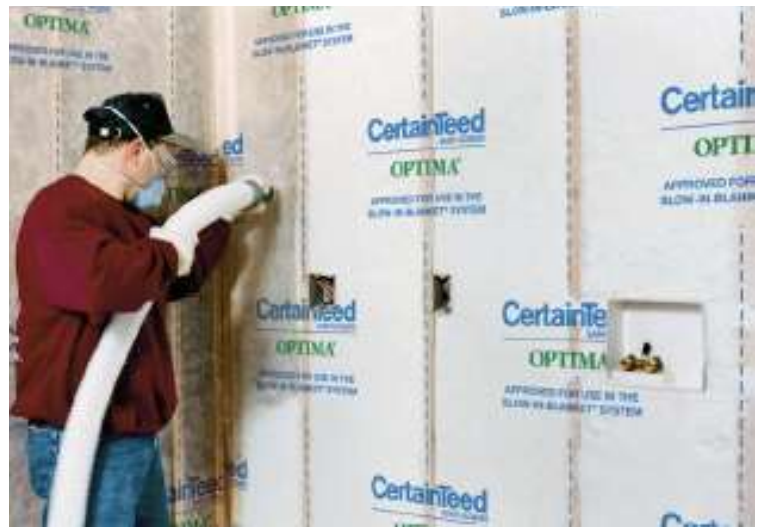
Figure 3: Installation of blowing wool in closed cavity application
