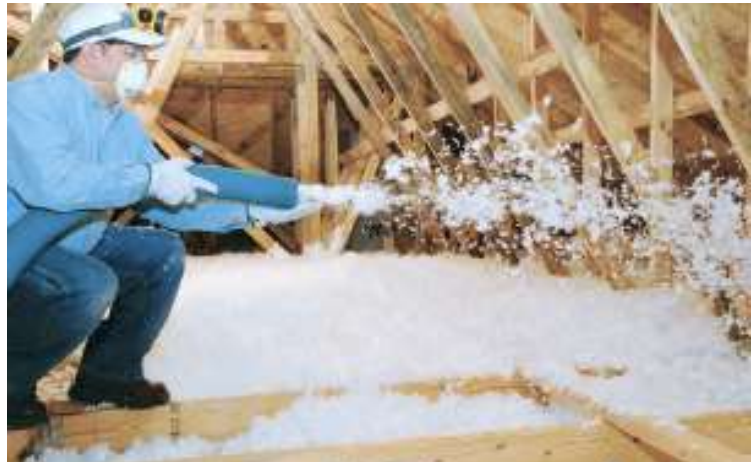
Figure 2: Installation of blowing wool in open cavity application
