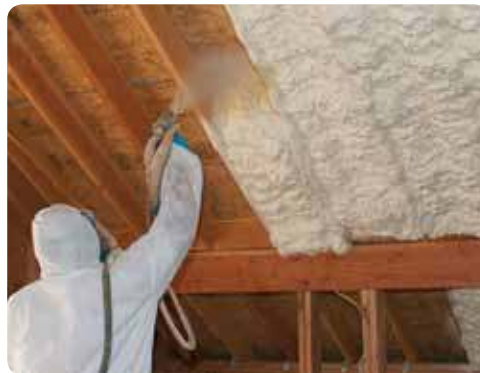
Spray Foam Insulation
