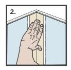
Press LEVELLINE trim into position and straighten.
