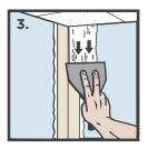
Using a 4" finishing knife, remove excess mud and let dry.
