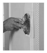
Outside corners. Using a 6" knife, apply the first coat of joint compound along one flange of the corner bead and smooth the compound outward with the knife. Repeat the process on the other flange. Allow the compound to dry and repeat the process again, using a 10" knife, feathering the edges outward.
