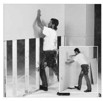
Glue. Even strong constructiongrade panel adhesives must be reinforced with nails and screws. Make sure the framing surfaces are clean and free of contamination. Apply adhesive, following the manufacturer's instructions. Then use nails or screws, spacing them 16" apart in the field of the boards.
