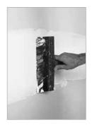
**Finishing coat.** Scrape, sand or use a damp sponge to gently remove any imperfections. Draw a 10" knife blade along the surface to ensure it is level. Apply a thin finishing coat to each joint, then feather outward 3" to 4" to eliminate imperfections.
