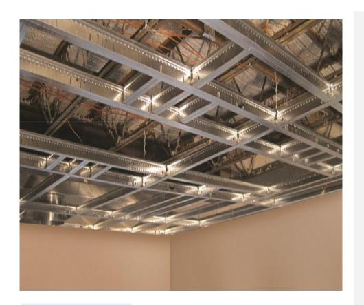
Acoustic ceiling and drywall suspension systems with a range of aesthetic and performance properties.
