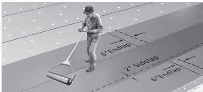
Figure 5-15: Roll seams with a heavy weighted roller.
