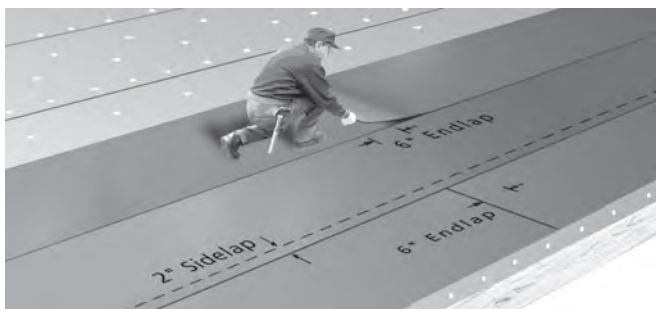
Figure 5-16: Overlap sidelaps of Mid Ply or PlyBase.
