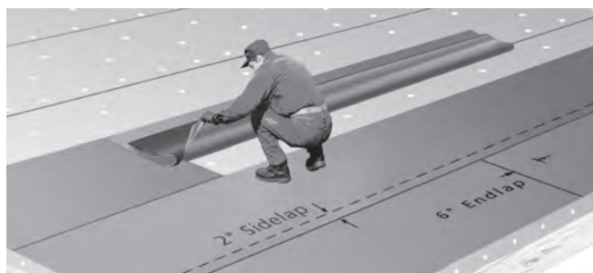
Figure 5-14: Fold membrane back halfway and remove release film.
