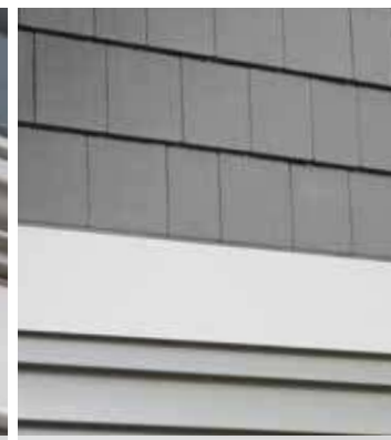
Band Board with foam insert can create a transition between two siding styles.
