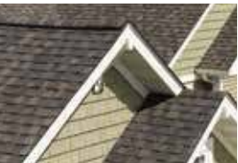
ROOFING AND VENTILATION
