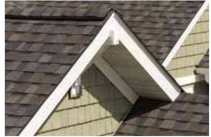
ROOFING AND VENTILATION
