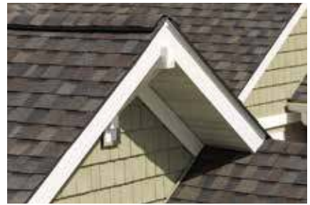
ROOFING AND VENTILATION
