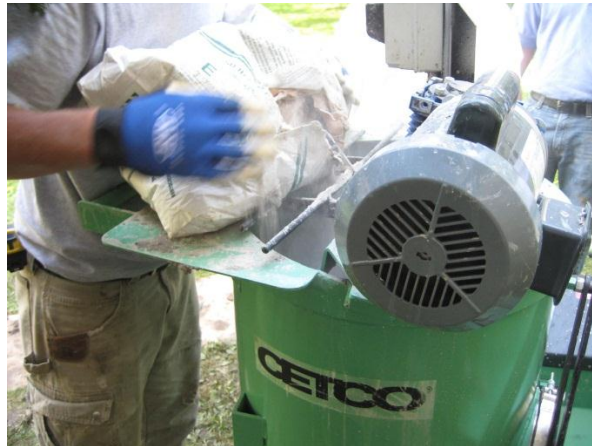
Utilizing the forks on the covering grate to open BentogROUT bag.
