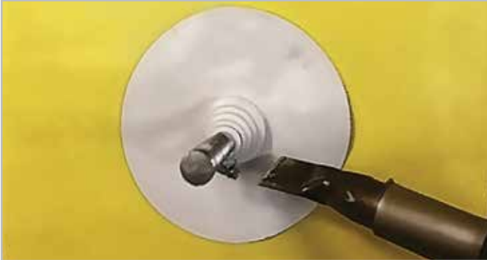
STEP 7. Hot-air applied to stepped stack
