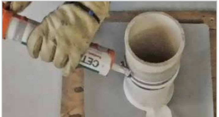
STEP 9. Apply CETSEAL bead at termination
