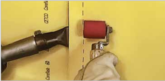
STEP 2. Pre Weld Placement
