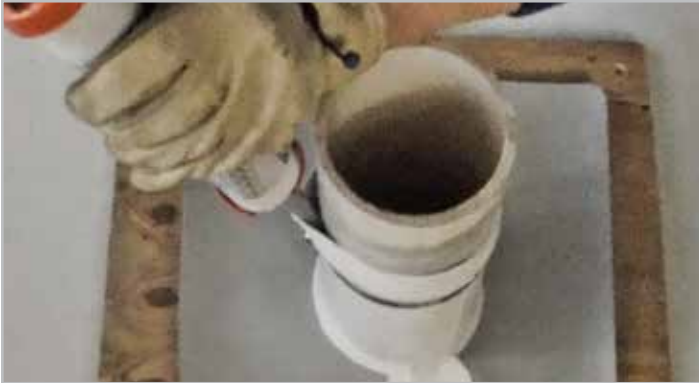
STEP 6. Install AKWASWELL bead
