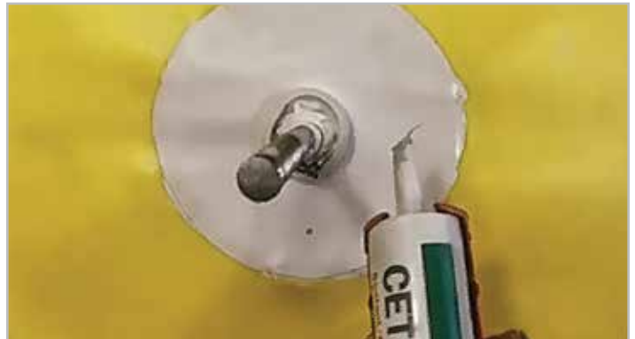
STEP 10. Apply CETSEAL at termination
