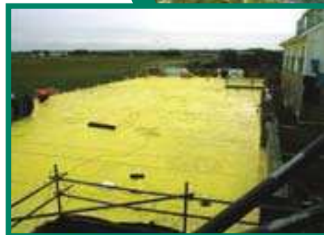
Greenroof under construction with COREFLEX® waterproofing system
