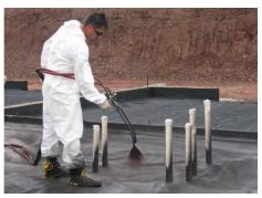
LIQUID BOOT® 500 spray-application effectively seals penetrations, footings, grade beams and other irregular surfaces that are considered critical vapor intrusion pathways.
