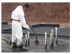
In addition to superior chemical resistance performance, LIQUID BOOT® sprayapplication effectively seals penetrations, footings, grade beams and other irregular surfaces that are considered critical vapor intrusion pathways.
