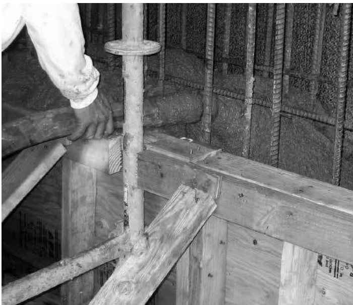
Photo H3-3: SHOTCRETE PLACEMENT IN KICKER FORM Apply project approved shotcrete mix without air velocity into minimum 600 mm (24 inch) high kicker form and then consolidate by vibration
