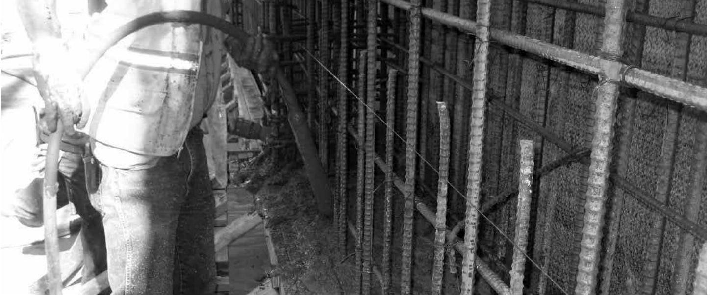
PHOTO 1: KICKER FORM AT BASE OF SHOTCRETE WALL
