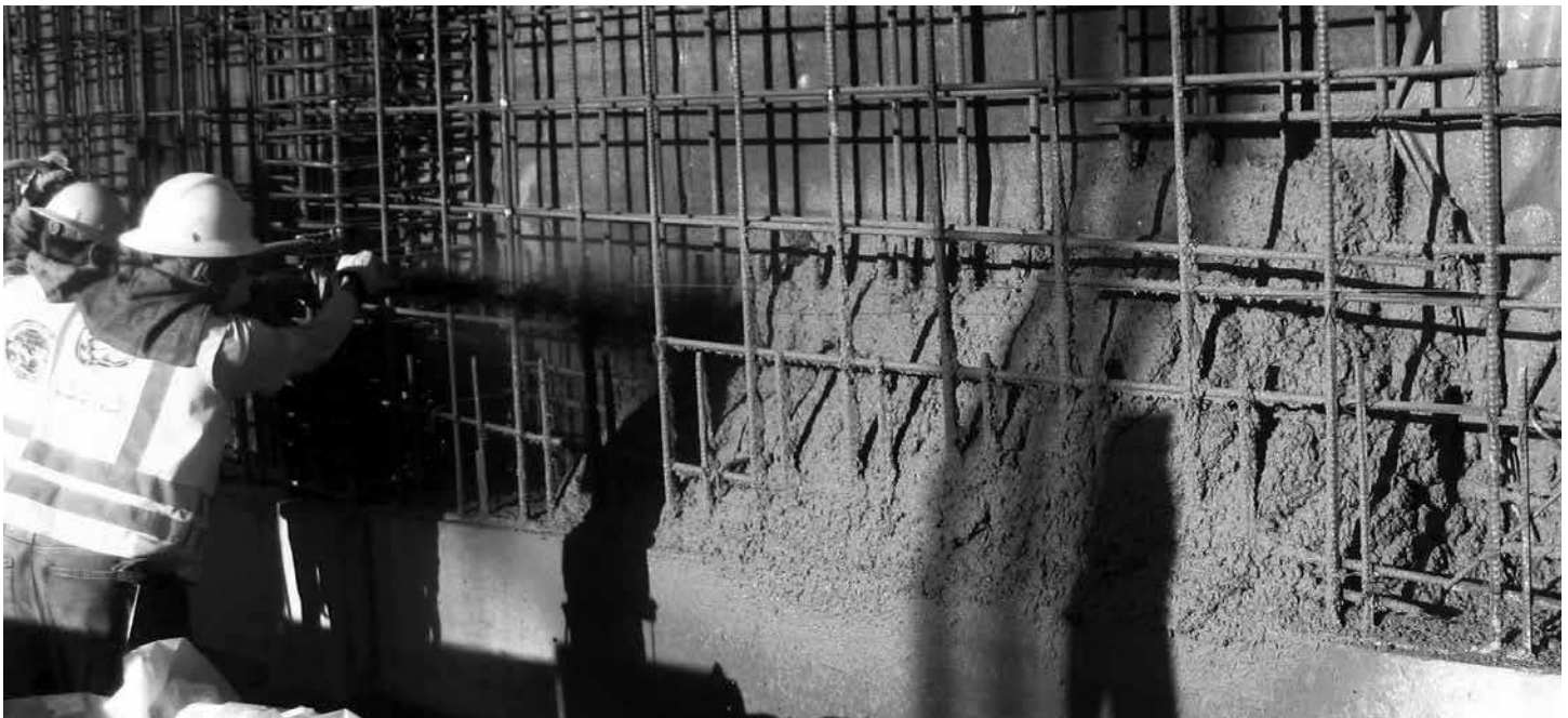
PHOTO 2: SHOTCRETE FOUNDATION WALL
