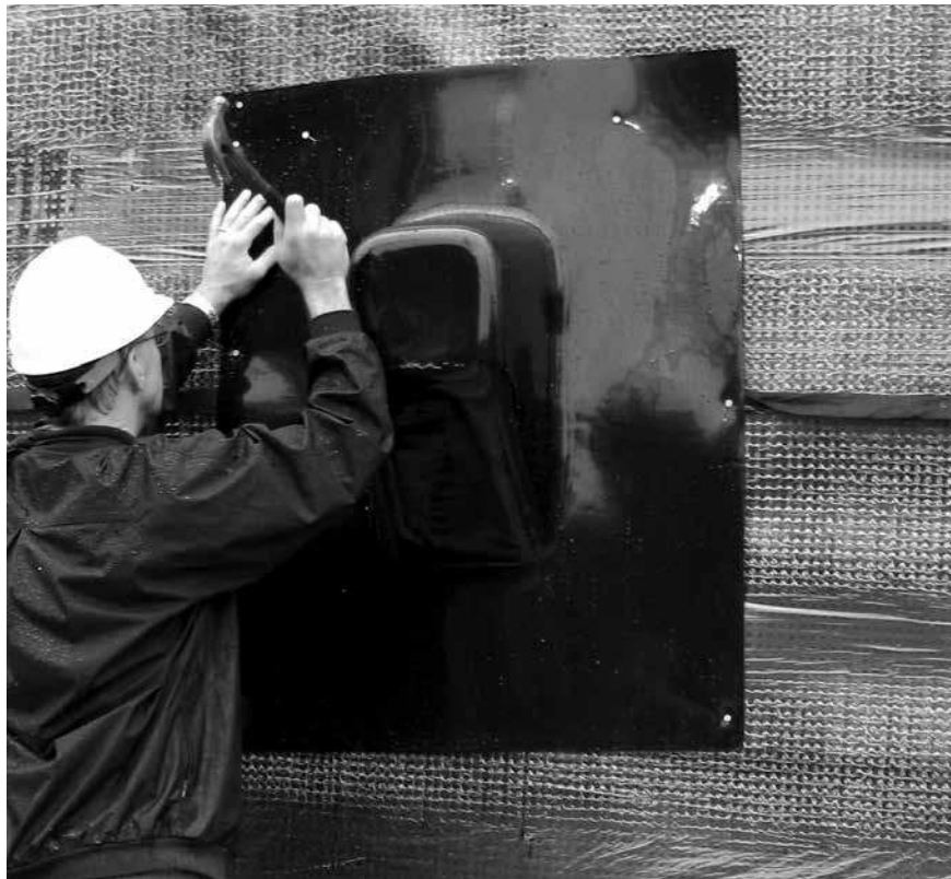
PHOTO 6: TB-BOOT (NON-HYDROSTATIC)
