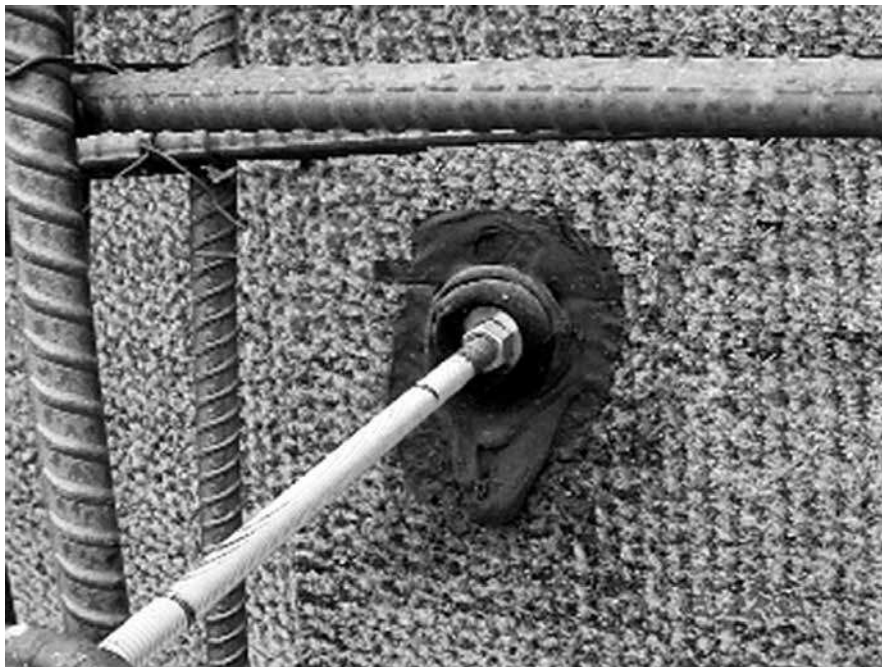
PHOTO 4: REBAR ANCHORAGE DETAILING
