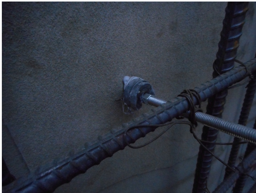
PHOTO 2: REBAR ANCHORAGE DETAILING
