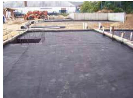
ULTRASHIELD™ G-800 is a needle-punched, non-woven geotextile with superior tensile strength and puncture resistance.
