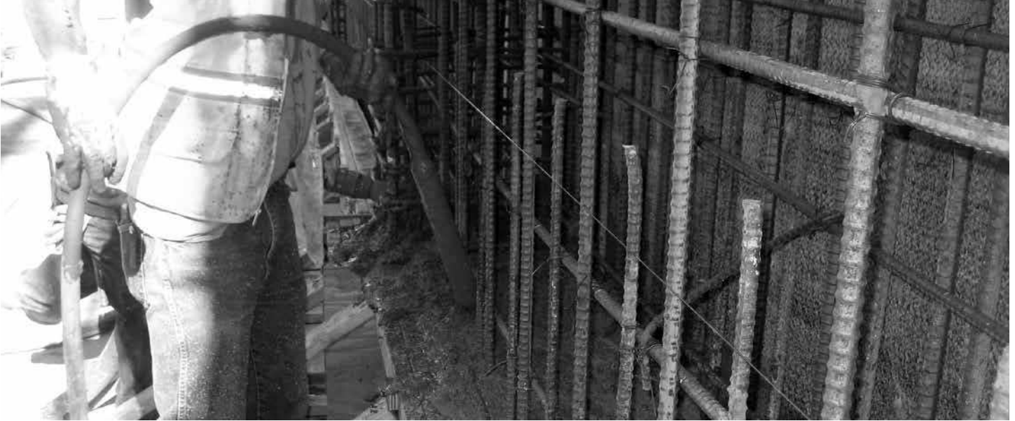
PHOTO 1: KICKER FORM AT BASE OF SHOTCRETE WALL
