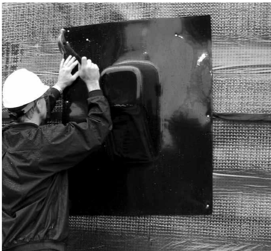
PHOTO 6: TB-BOOT (NON-HYDROSTATIC)
