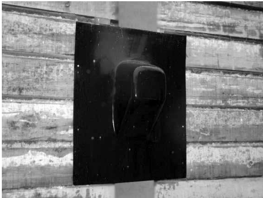
PHOTO 5: TB-BOOT OVER (HYDROSTATIC)
