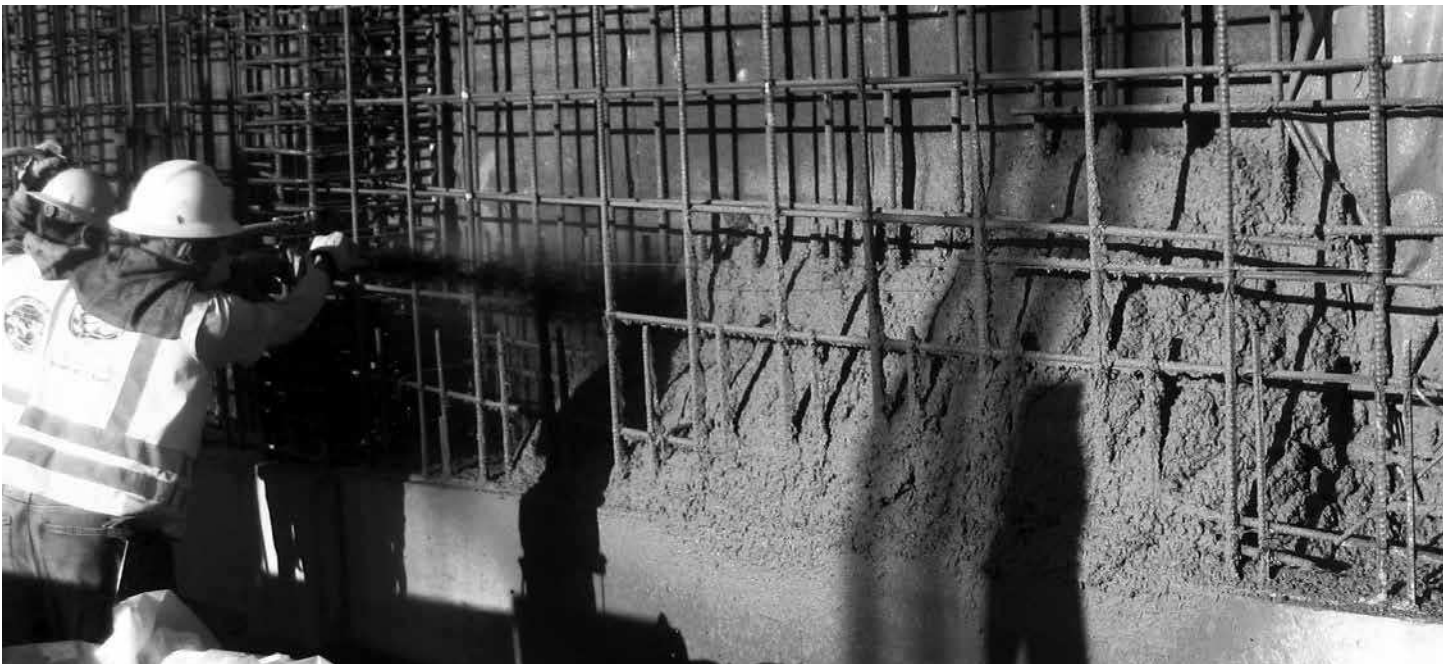
PHOTO 2: SHOTCRETE FOUNDATION WALL
