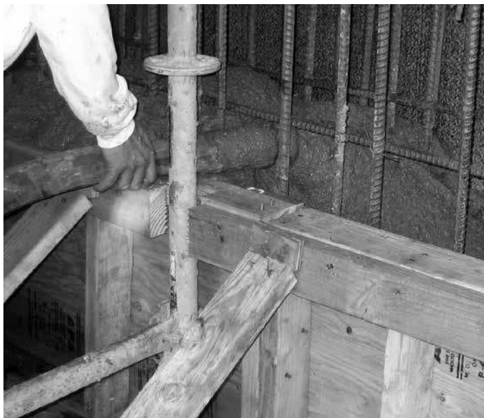
Photo H3-3: SHOTCRETE PLACEMENT IN KICKER FORM
