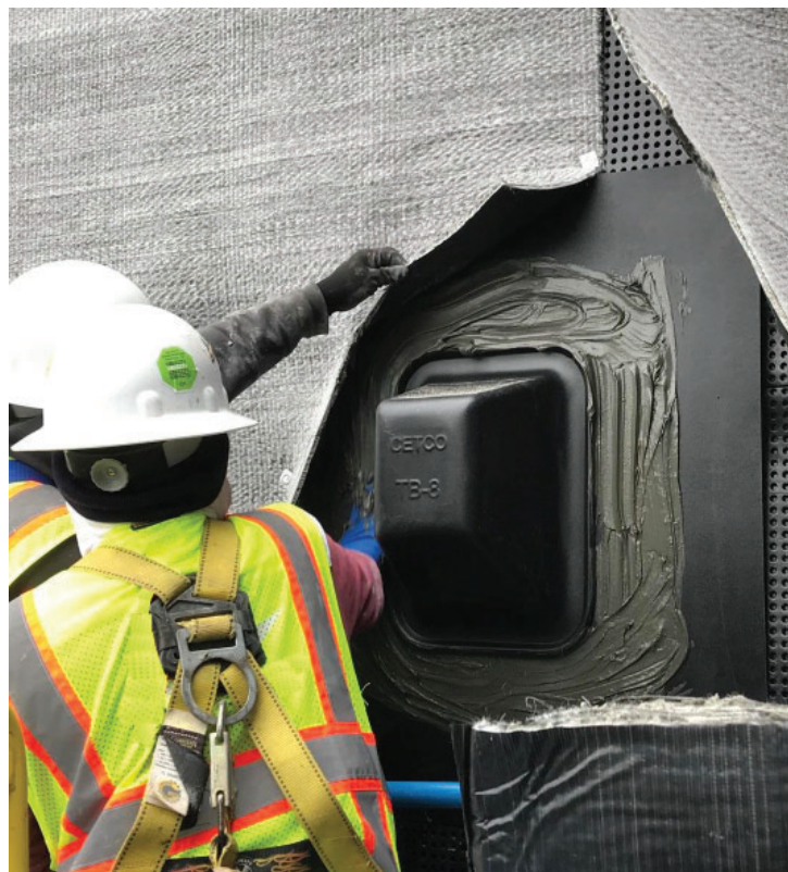
PHOTO 4: TB-BOOT (NON-HYDROSTATIC)
