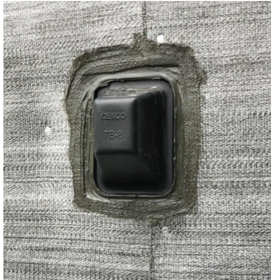
PHOTO 3: TB-BOOT OVER (HYDROSTATIC)
