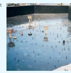
Focal point water features often require linings to adhere to and bridge between stainless steel, copper, CMU, concrete and PVC protrusions, withstand intense UV conform to complicated shapes, and allow short construction windows.
