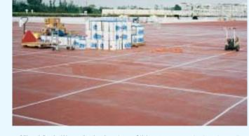
Miami-Dade Water Authority chose CIM 1061 to coat the interior walls and CIM 1000 to coat the roof deck of their new 20-million gallon potable water reservoir. The reason: CIM's ANSI/NSF certification, and the product's ability to bridge cracks and withstand structural movement.
