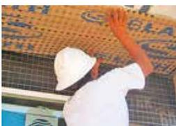
V Truss® for walls and ceilings was designed by Structa Wire Corp to improve the performance of stucco on overhead surfaces. This self-furring, welded wire lath is also approved for use on vertical surfaces and as a reinforcing component for rainscreen wall systems.
