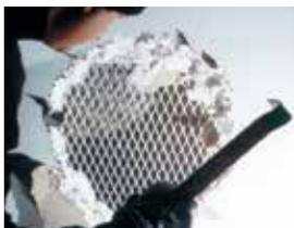
This tough, rigid heavy-gauge security mesh is used behind common-wall substrates to protect against break-ins and break-outs. Tough to smash or cut, it safeguards walls and ceilings in homes, apartments, offices, stores, vaults, storage areas and correctional facilities. Also fire-resistant, barrier mesh is a cost-effective, time-saving alternative to reinforced concrete or concrete block.
