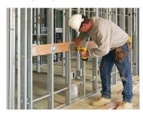
Secure each plate to the stud flange using two small pan or wafer-head screws.
