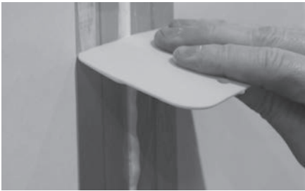
FIGURE 18: REMOVING EXCESS SEALANT
