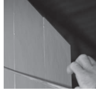
FIGURE 20: REMOVING PAINTER'S TAPE
