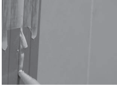
FIGURE 19: BUMP ADHESIVE IN TO PREVIOUS SECTION
