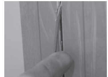
FIGURE 12: REMOVE EXCESS ADHESIVE
