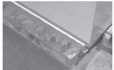
FIGURE 22: HORIZONTAL SEAM FILLED COMPLETELY WITH SEALANT
