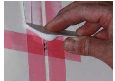
Figure 17: Applying the painter tape horizontal in 3' sections
