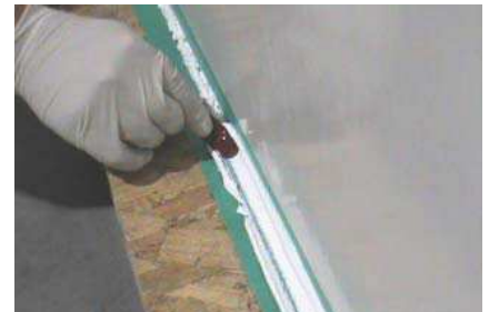
Figure 23: Horizontal finish with rounded corner
