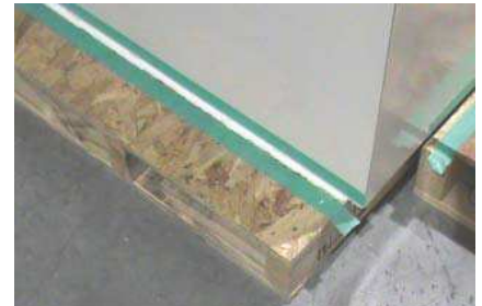
Figure 22: Horizontal seam filled completely with sealant
