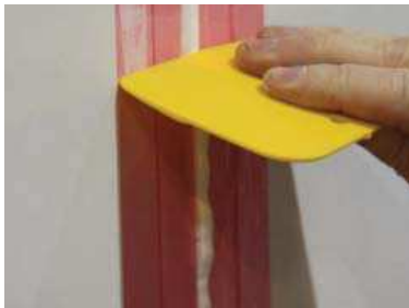
Figure 18: Removing excess sealant
