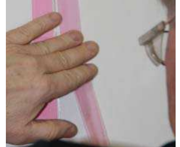
Figure 16: Applying the painter tape
