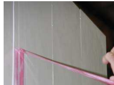
Figure 20: Removing Painter's tape
