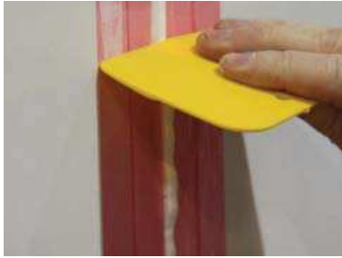
Figure 18: Removing excess sealant
