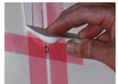
Figure 17: Applying the painter tape horizontal in 3' sections
