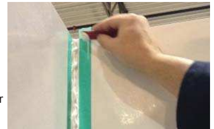
Figure 21: Using Radial Seam Finisher for rounder corner joint
