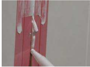
Figure 19: Bump adhesive in to previous section
