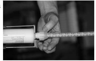
FIGURE 14: ATTACH STATIC MIXING TIP
