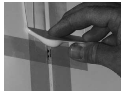
FIGURE 17: APPLYING THE PAINTER TAPE HORIZONTAL IN 3' SECTIONS
