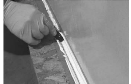
FIGURE 23: HORIZONTAL FINISH WITH ROUNDED CORNER
