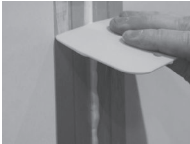
FIGURE 18: REMOVING EXCESS SEALANT
