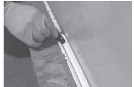
FIGURE 23: HORIZONTAL FINISH WITH ROUNDED CORNER
