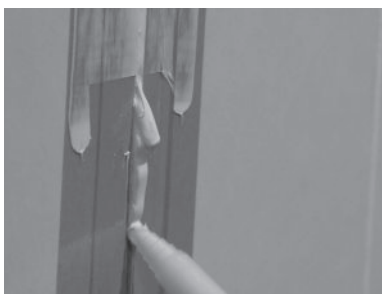
FIGURE 19: BUMP ADHESIVE IN TO PREVIOUS SECTION
