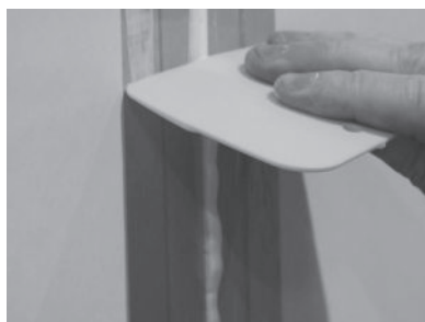
FIGURE 18: REMOVING EXCESS SEALANT
