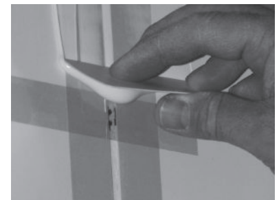
FIGURE 17: APPLYING THE PAINTER TAPE HORIZONTAL IN 3' SECTIONS
